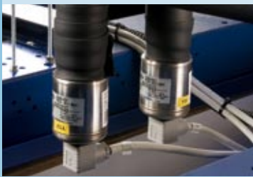
Electronic thermostatic expansion valves
